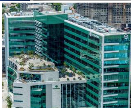
Old Mutual Sandton Supply & Install Access Flooring
