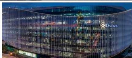
Discovery Health Sandton Supply & Install Access Flooring
